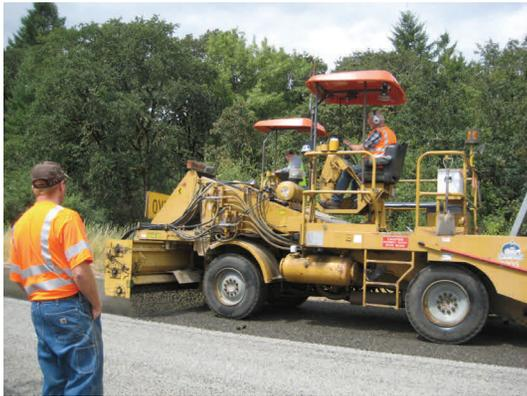
**T**his summer, Public Works crews will refurbish several of county roads with a new layer of gravel and emulsified asphalt. This process, called chip sealing, is done annually on various roads throughout the County. The treatment extends the life of each road by seven to ten years and provides a new sealed surface, at a fraction of the cost of a standard asphalt overlay.
