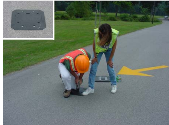
Figure 10-2 Electronic Vehicle Counter Installation (1)
