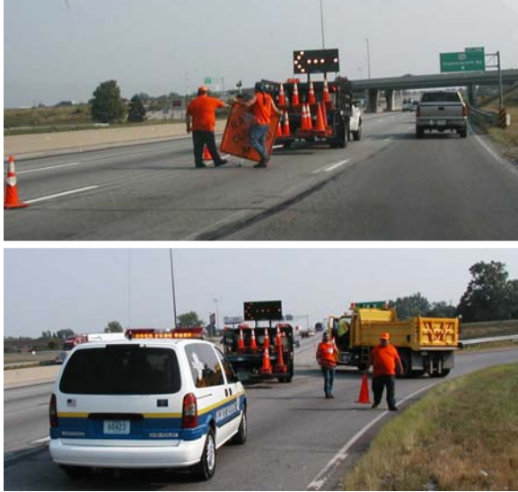
Figure 6-39 Temporary Elimination of Freeway Weaving Area
