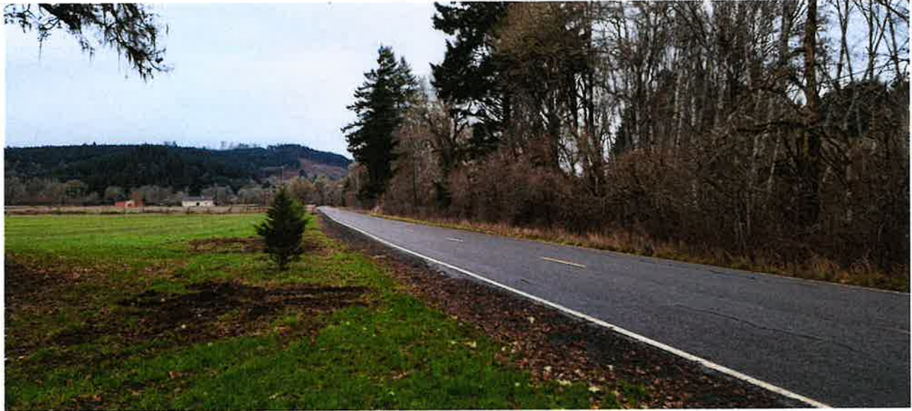
Figure 2 A– Site Access on Gold Creek Road (Looking North – Over 1,000 Feet Line of Site)
