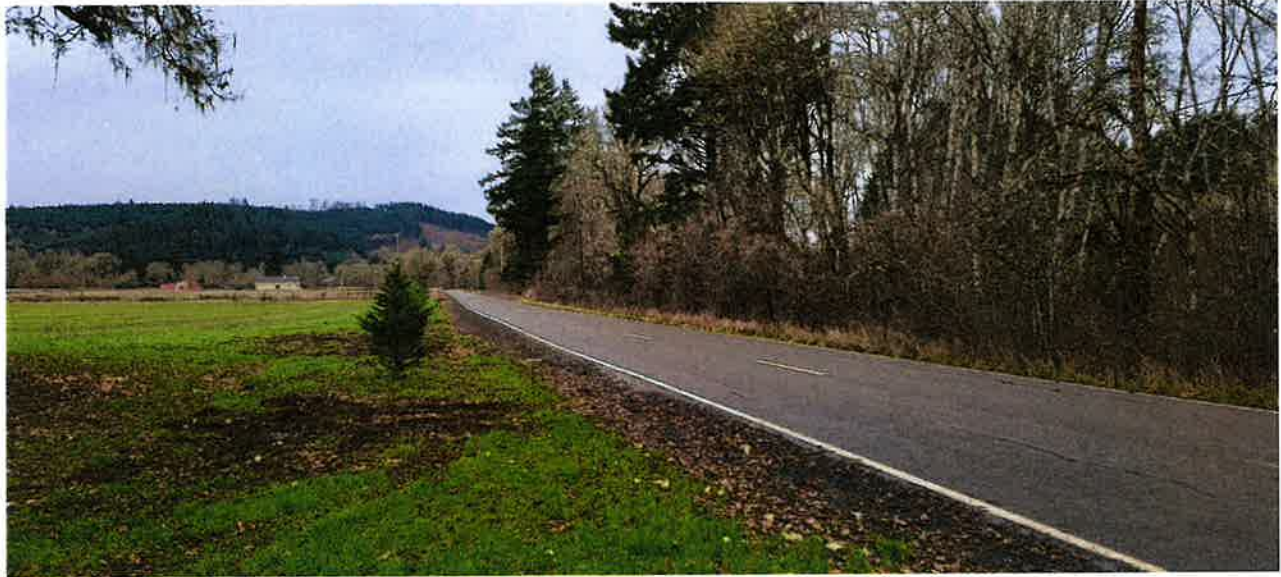
Figure 2 A– Site Access on Gold Creek Road (Looking North – Over 1,000 Feet Line of Site)
