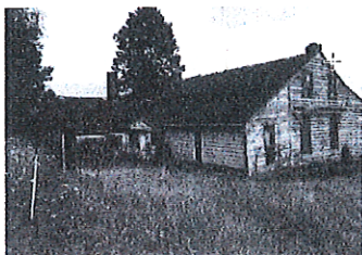
Figure 16: Existing south facing side of the Phillips House.
