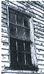
Figure 3: Existing window type on the north and south sides.
