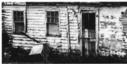
Figure 10: Existing windows on the north elevation of the existing addition
