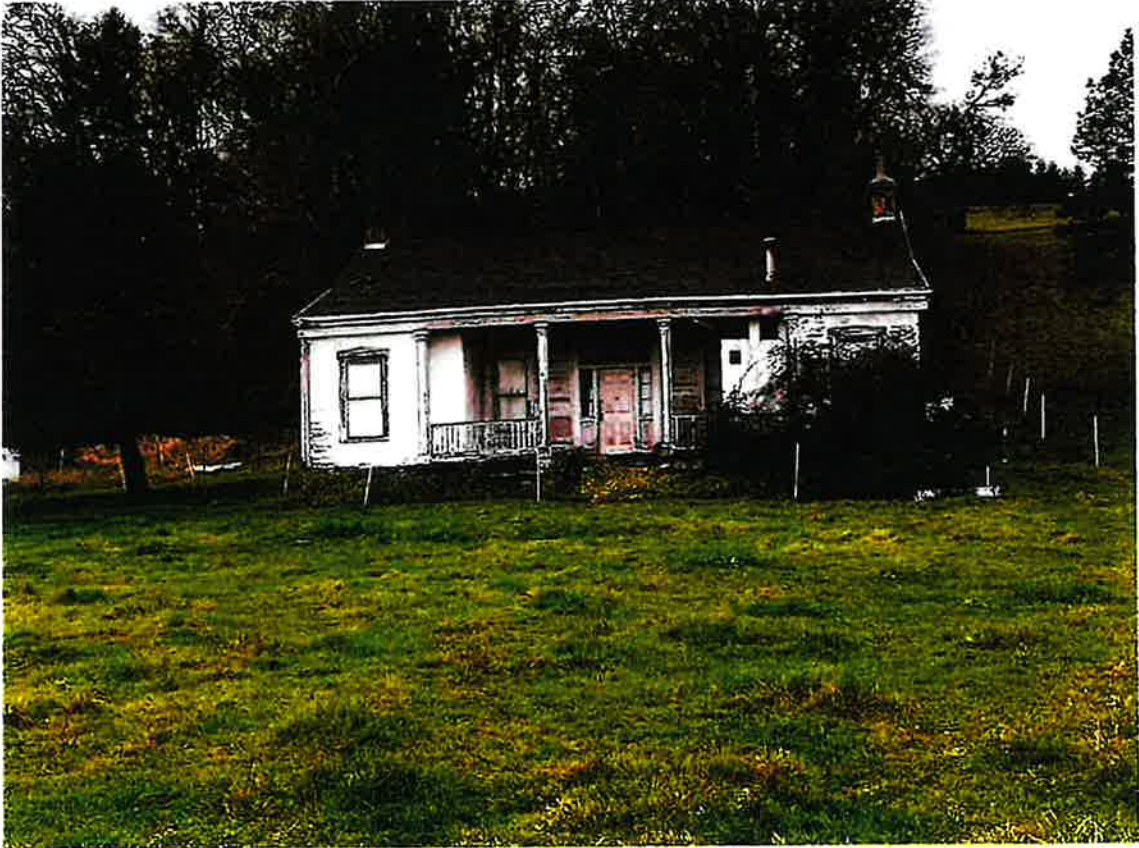
Figure 1- East Side of House, Front/ View from Road
