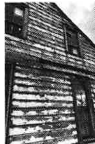
Figure 4: Existing window types on the south elevation (attic and parlor room)
