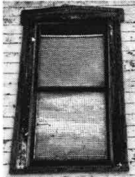
Figure 1: Existing windows on the east elevation (front) of the Phillips House.
