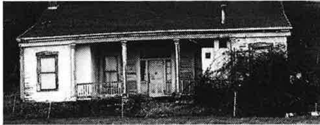
Figure 14: Existing east facing side (front porch) of the primary dwelling.
