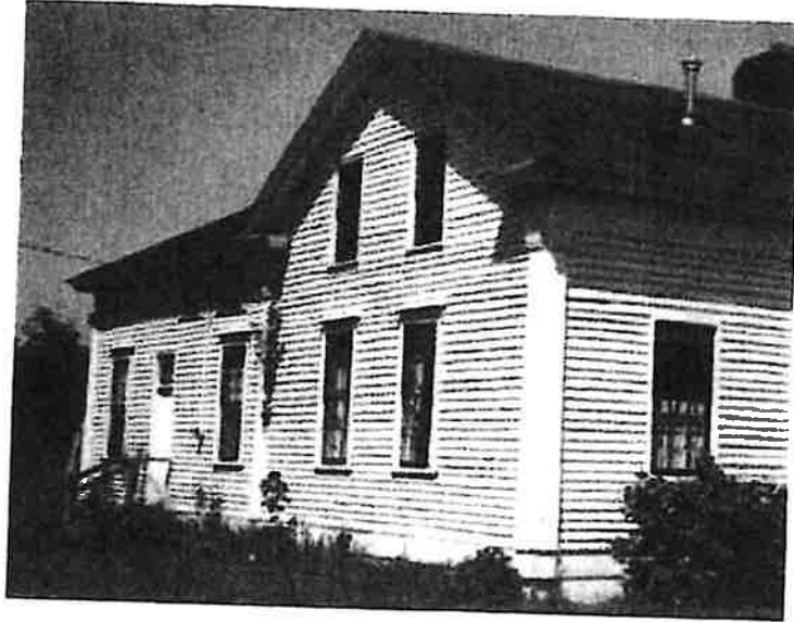
Jacob Conser House – Addition to the rear of the house with asymmetrical windows and smaller windows in the attic story, plus side door with uncovered stoop.
