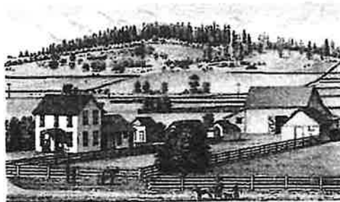
John Tait Farm, Lane County – Period lithograph shows a one-story rear addition with a shed-roofed porch and asymmetrical windows.
