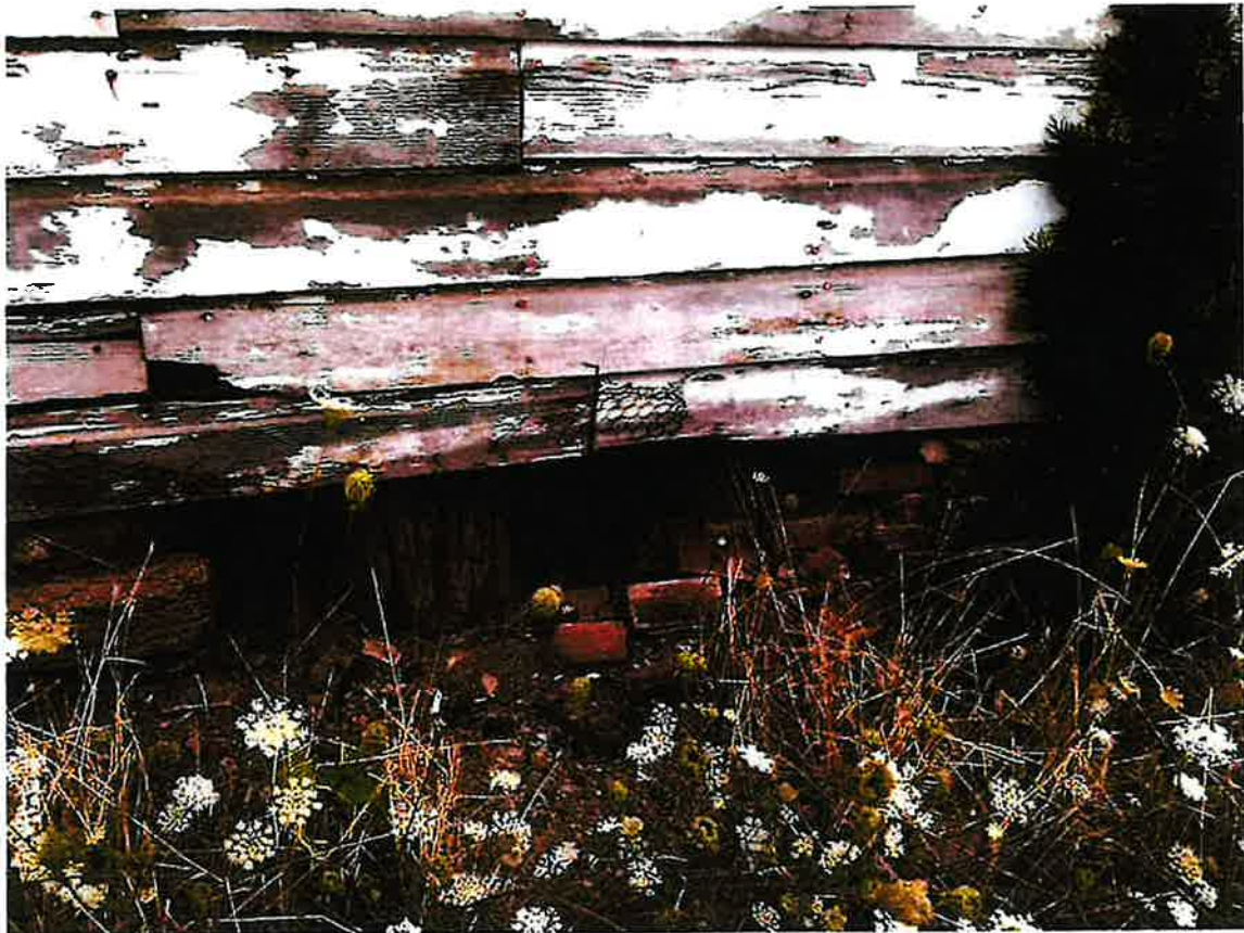
Figure 4- Foundation Beneath Original House to be restored
