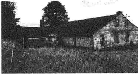
Figure 18: Existing south facing side of the Phillips House.
