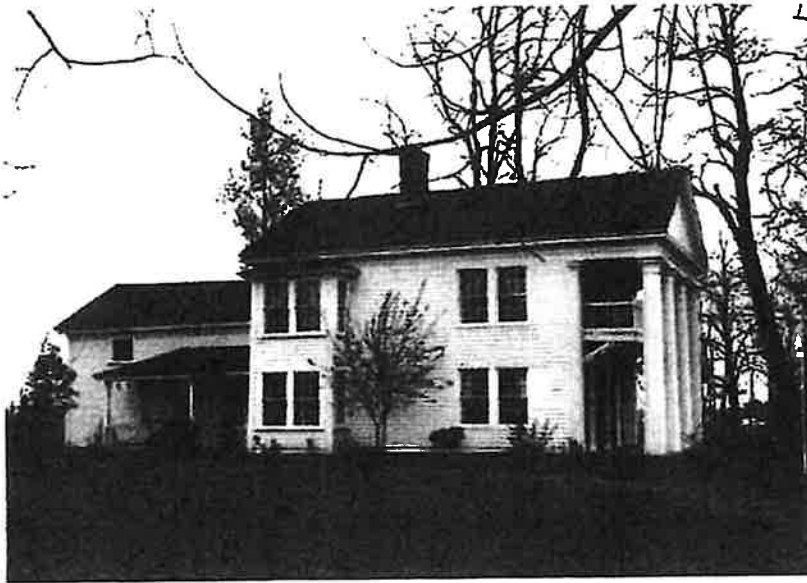
Opposite side of the John Ainsworth House, showing the rear addition with asymmetrical doors and windows. The very tall, almost French-door-like windows at the front porch can also be seen in this photo.
