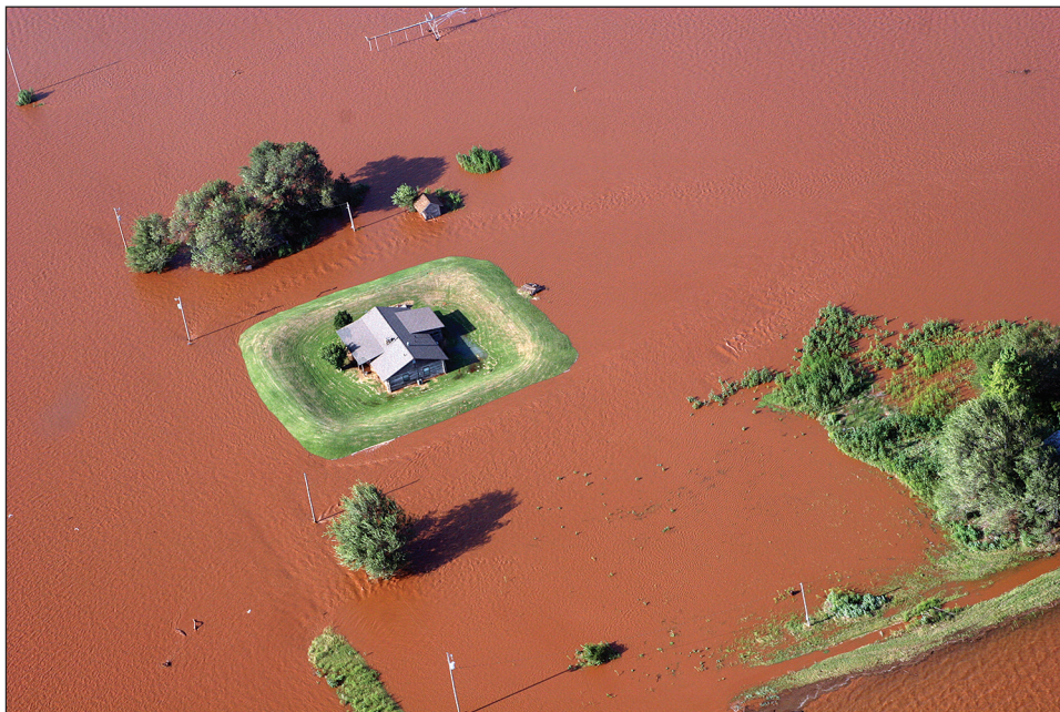
Figure 3-18. A home protected by a levee.
