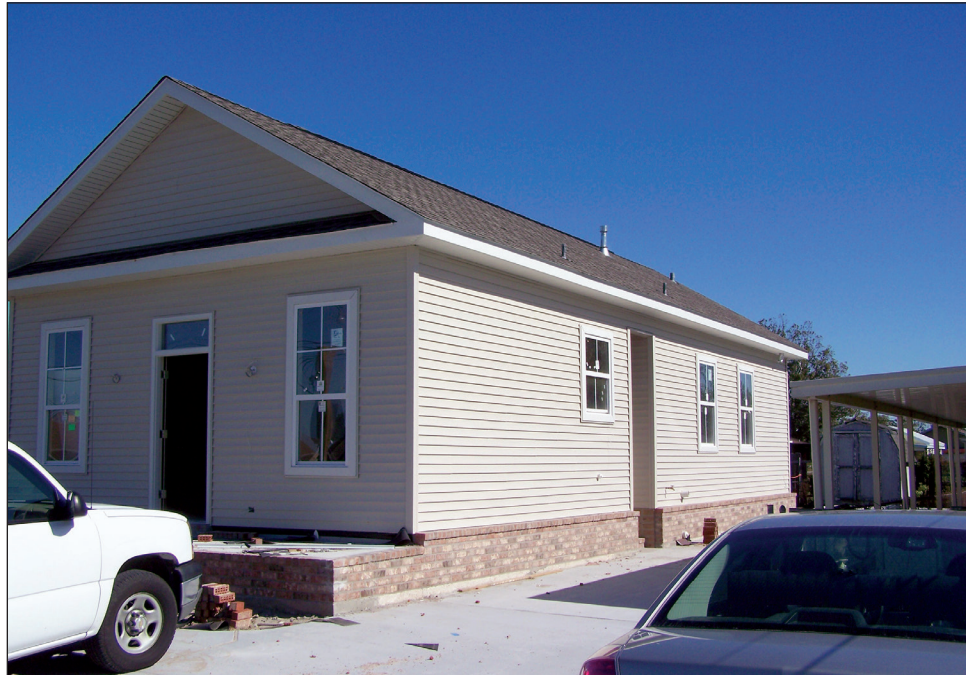
Figure 6-9. Typical mitigation reconstruction project.
