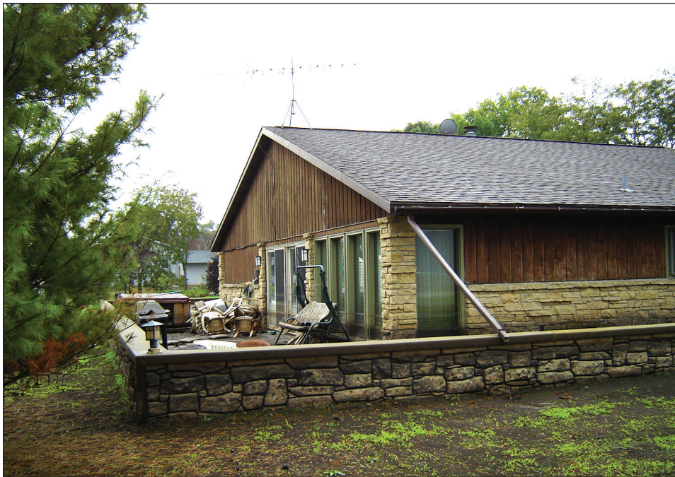
Figure 8-3. Structure protected by a floodwall with decorative stone finish.
