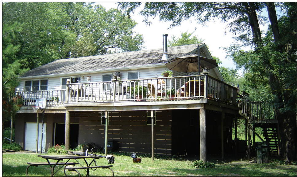
Figure 5-2. This home in Cedar Falls, IA, was elevated one full story. The garage and storage area are at the home's original elevation.
