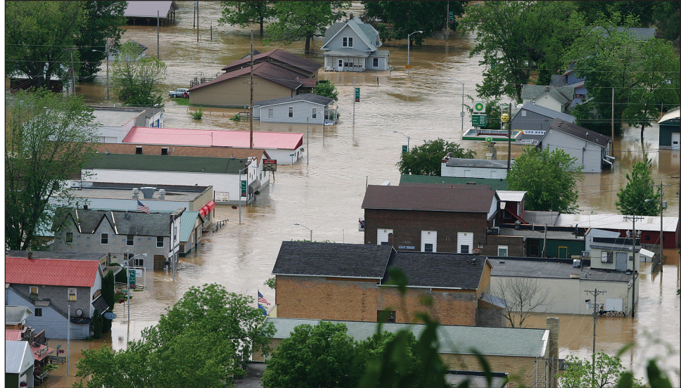
Figure 2-3. These homes in Gays Mills, WI, were inundated by riverine flooding during the Midwest floods of 2008.
