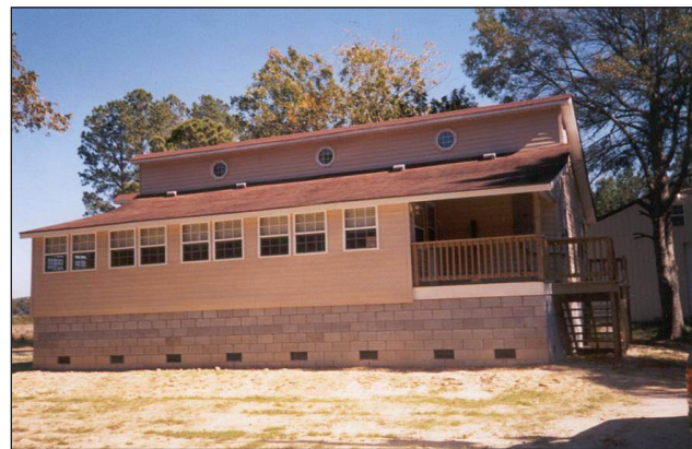
Figure 3-7. Before (left) and after (right) photos of a retrofitted home elevated on extended continuous foundation walls.
