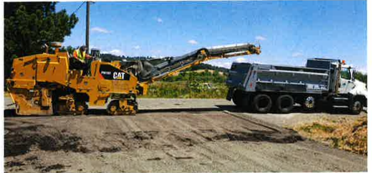
Road Crew members prepping a road approach for paving.
