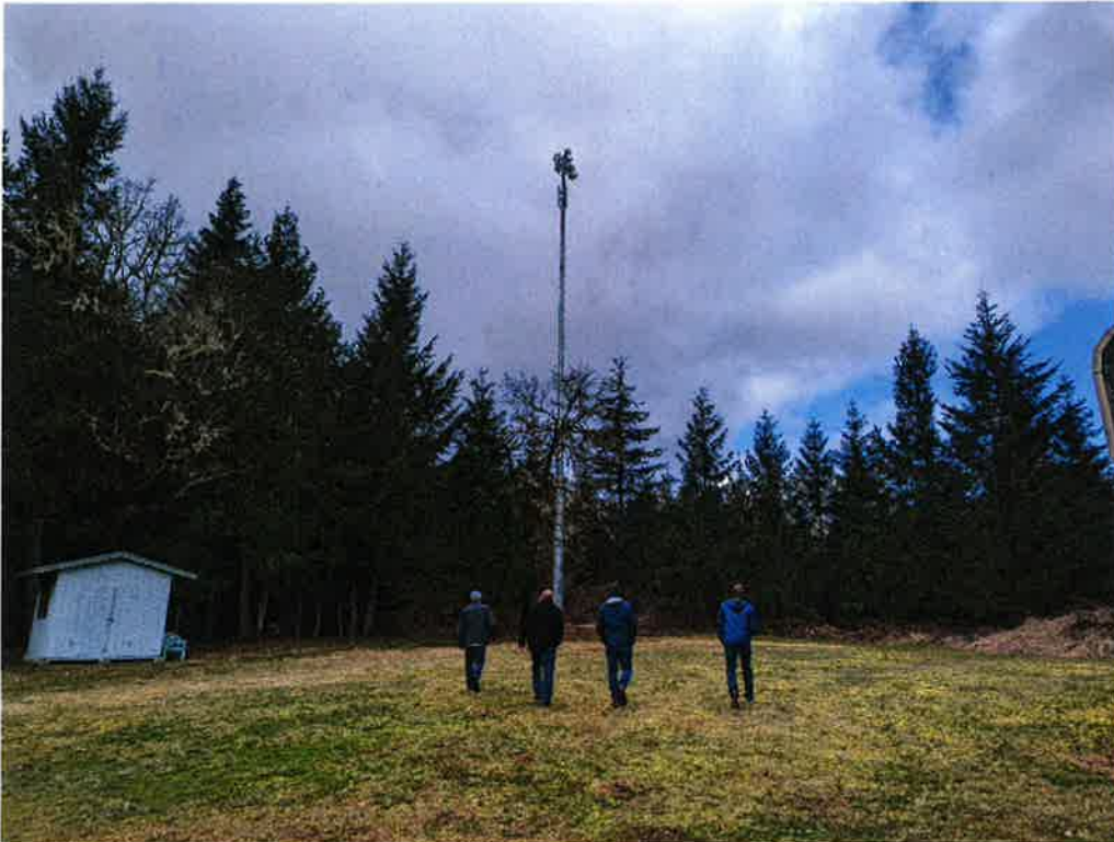
Alyrica CEO Sam Dotson and Polk County Commission Craig Pope (both pictured center) walk toward a newly constructed fixed wireless internet tower site north of Dallas, Oregon.
