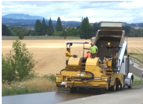
Road Crew members operating Chip Spreader
