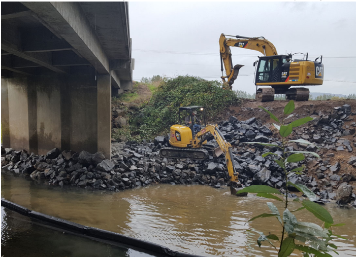
Erosion prevention project around a the base of a Polk County bridge.
