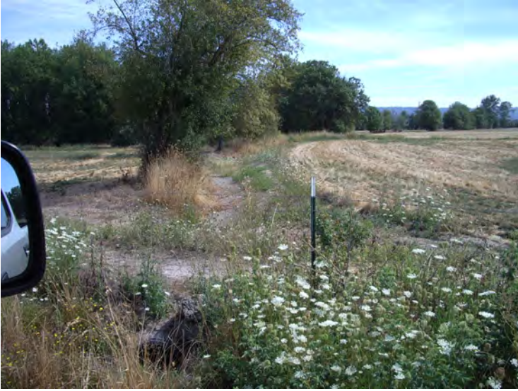
Site 23: Drainage ditch at culvert crossing (Station 617+00).
