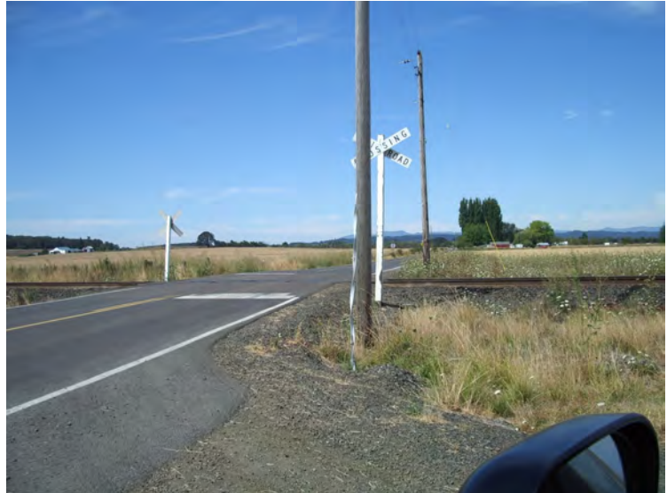
Site 21: SP Railroad crossing (Station 551+00).
