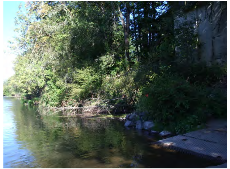
Site 1: Willamette River shoreline at existing intake structure.
