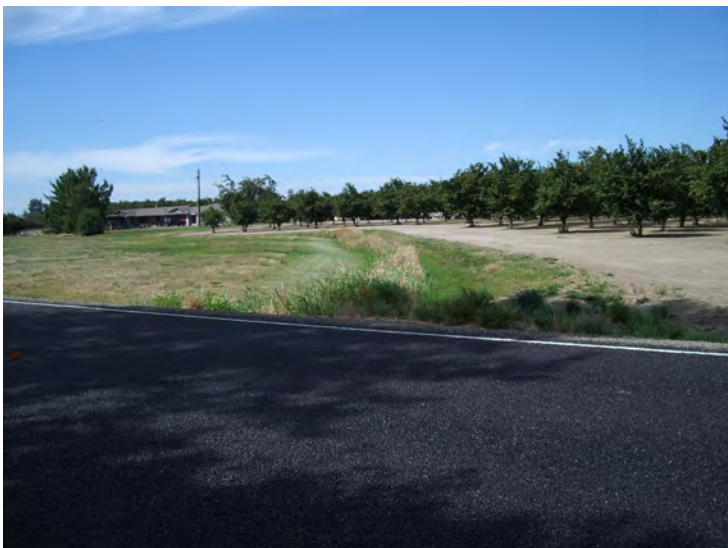
Site 16: Drainage ditch culvert crossing (Station (342+00)).
