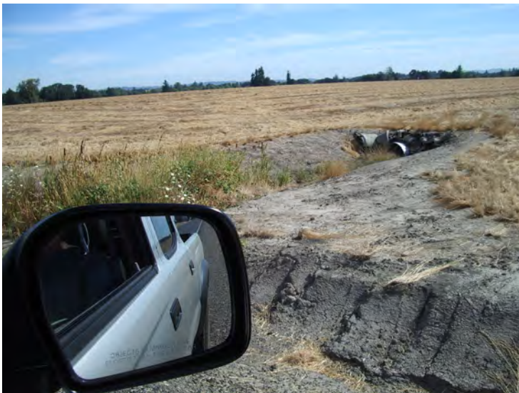
Site 13: Drainage ditch at Suver Road (Station 210+00).
