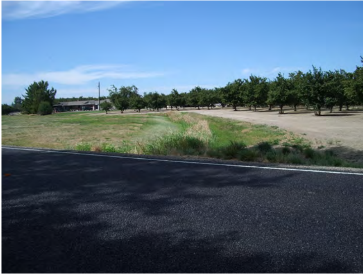
Site 20: Drainage ditch/emergent wetland at culvert crossing (Station 515+00).
