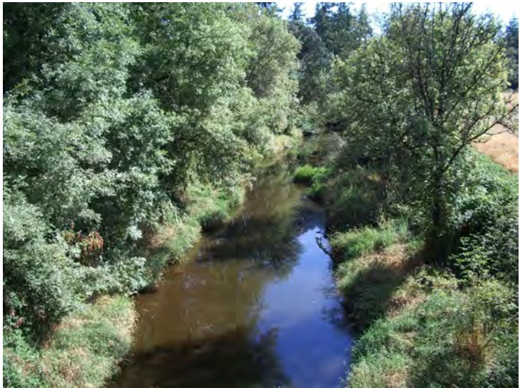
Site 12: Berry Creek bridge crossing (Station 143+00).
