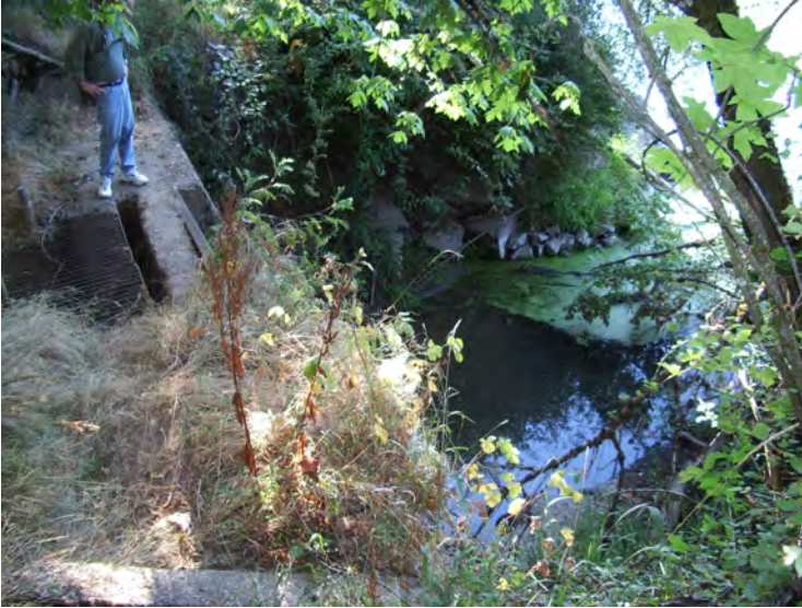
Site 1: Existing intake structure at Hyak Park (Station 00).
